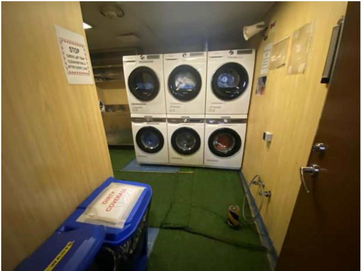
041. Laundry room main deck.
