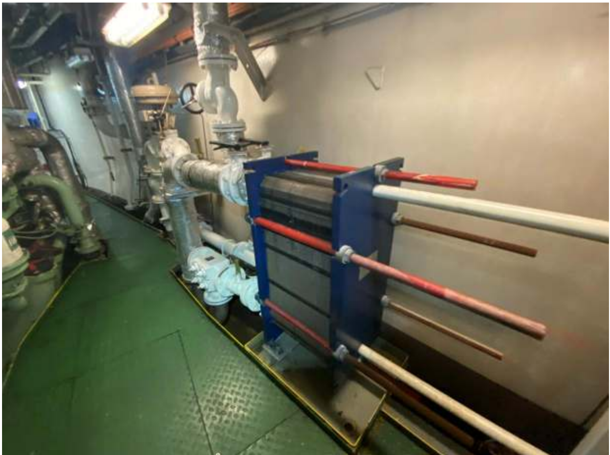
132. ME jacket cooler plate-type.
