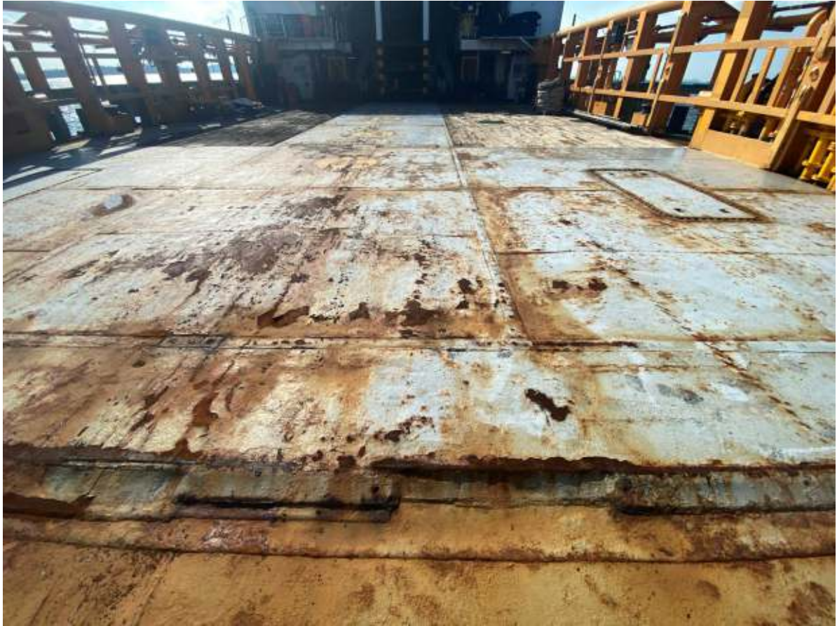
015. Main deck slightly in need of rust prevention and painting.
