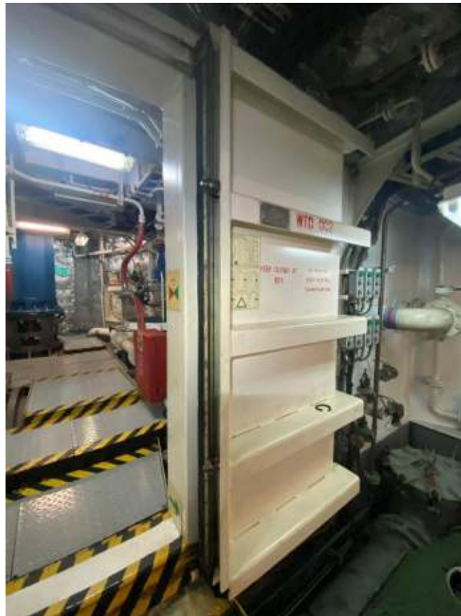
133. Watertight door leading into bow thruster room on lower space.
