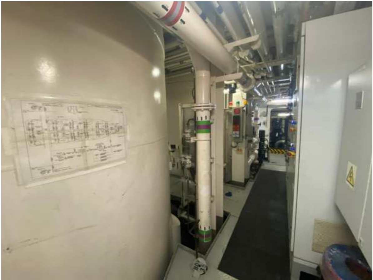
109. Mezz deck aft.
