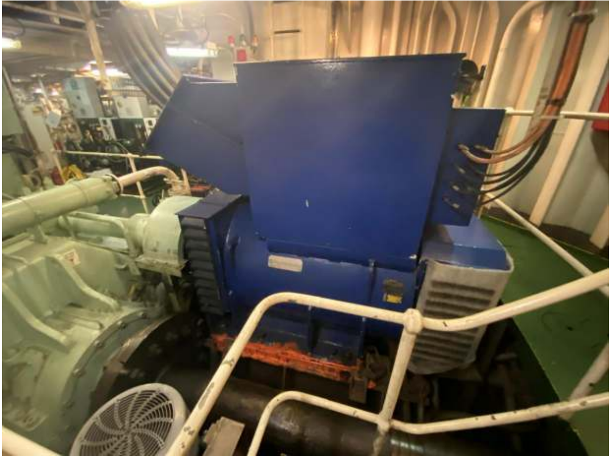
117. Electric propulsion motor.
