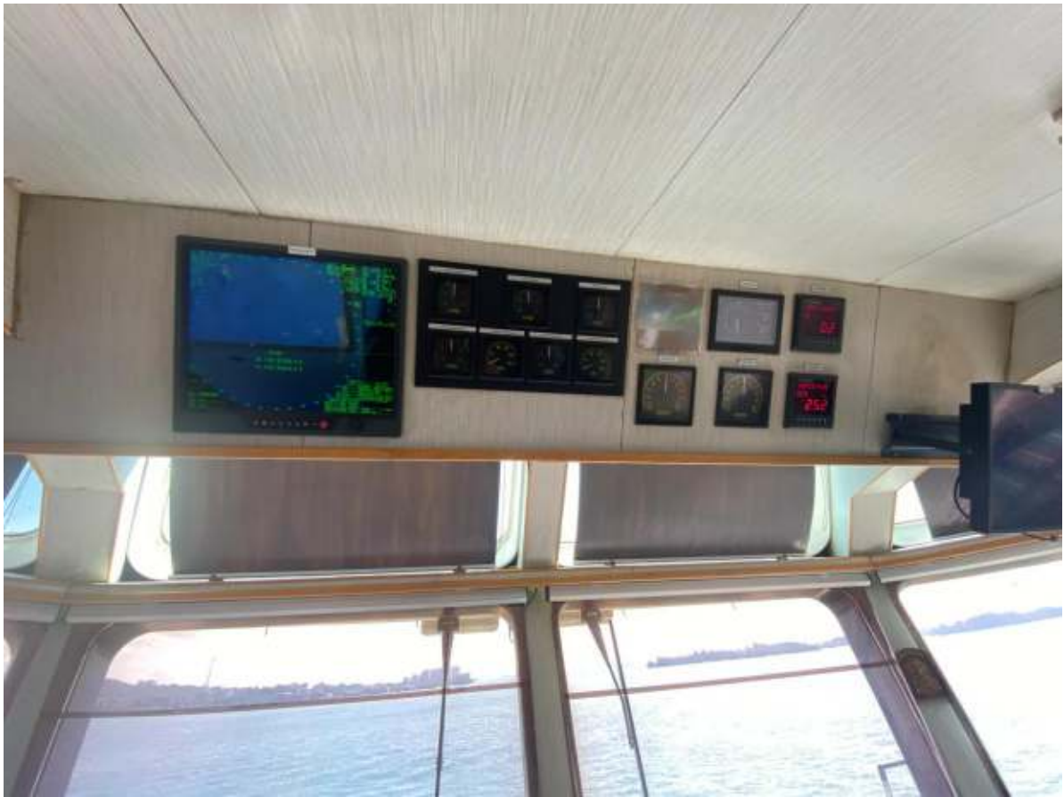
105. Radar and instrumentation panel.
