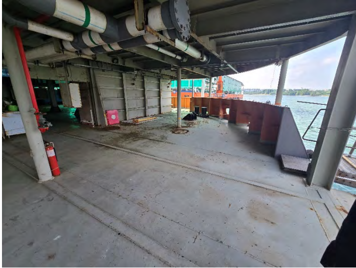
Forward main deck (P).
