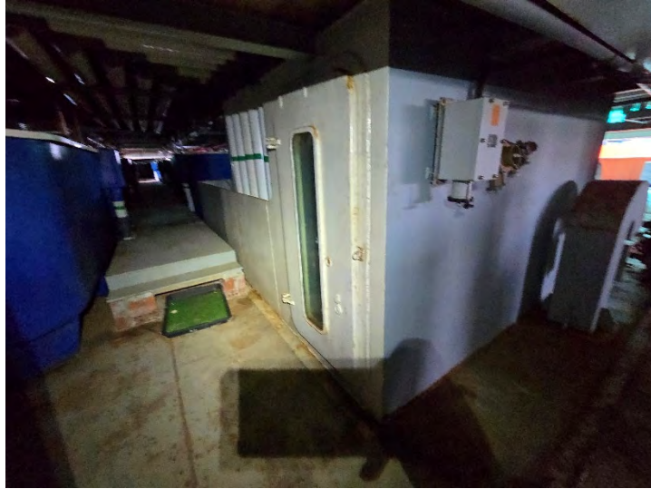
Accessway into below main deck.
