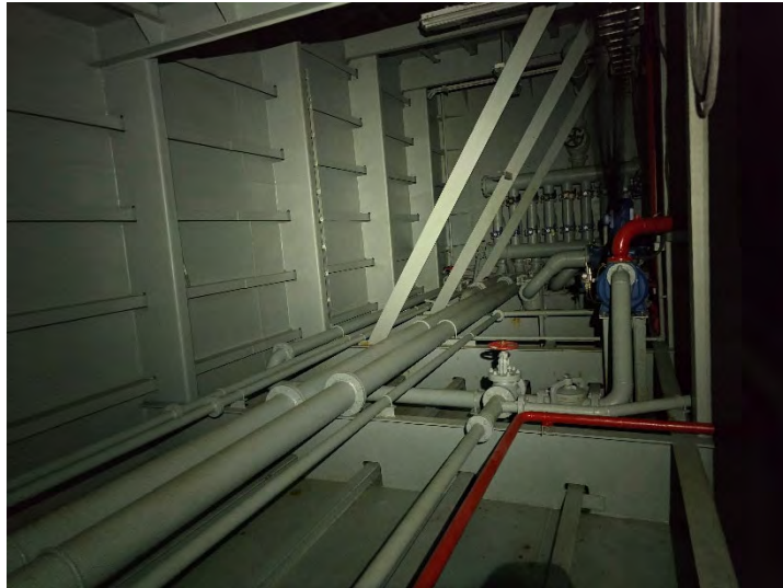
Below main deck space well coated and in good condition.
