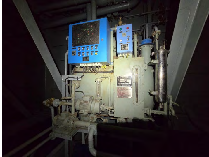
Sewage treatment plant.
