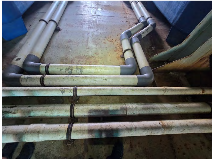
PVC piping appeared in good condition.
