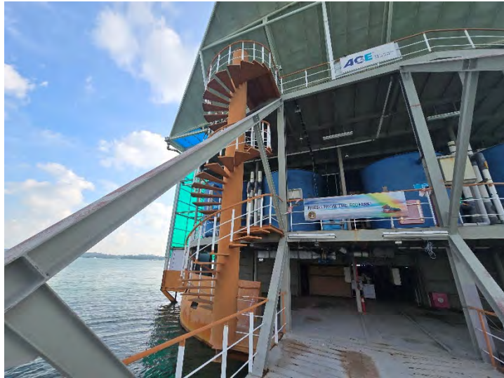
Spiral stairway accessing bridge deck mezzanine and main decks.
