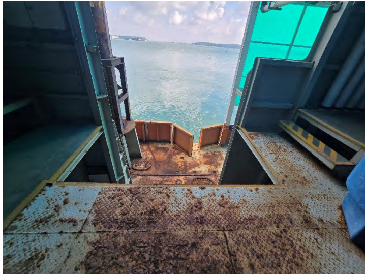
Mezzanine deck loading access starboard side.
