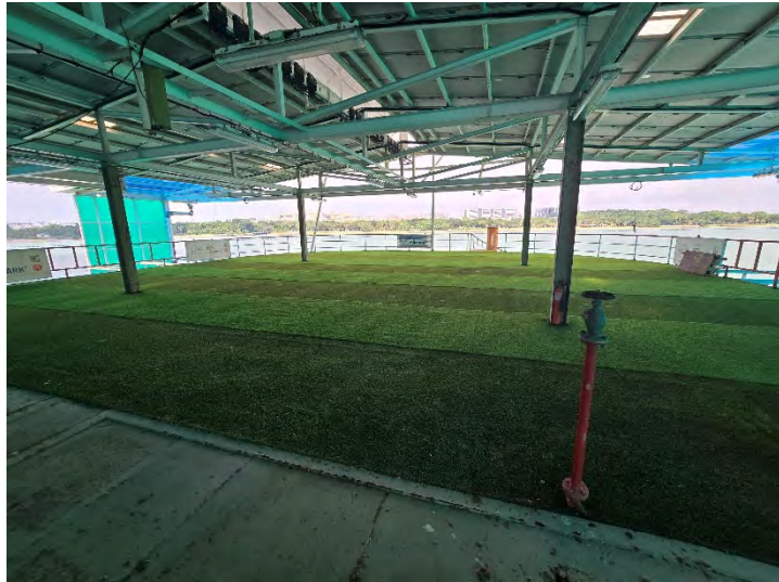
Faux grass section of the bridge deck.
